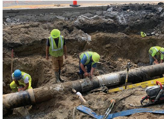
Water mains are designed to withstand the enormous force placed on them due to the frozen ground, but extended cold temperatures sometimes become too much for the main and they can break.
