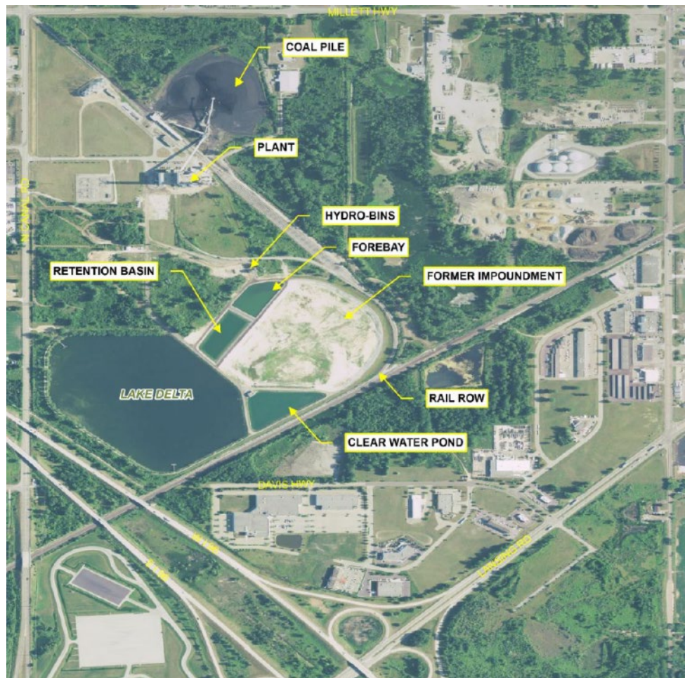
Figure 2. Erickson Power Station Site Configuration
